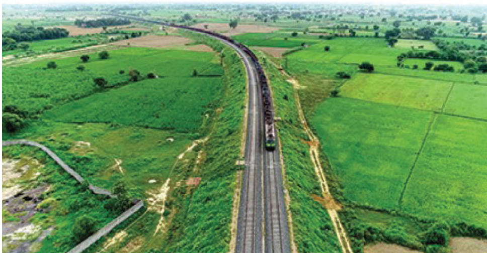
Photo: Goods train running on the eastern arm of Bhadan - Khurja section of Eastern dedicated freight corridor
