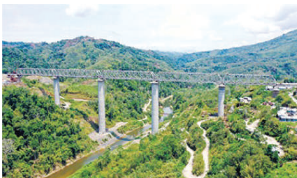
Photo: Jiribam-Imphal national railway project: bridge no. 44
