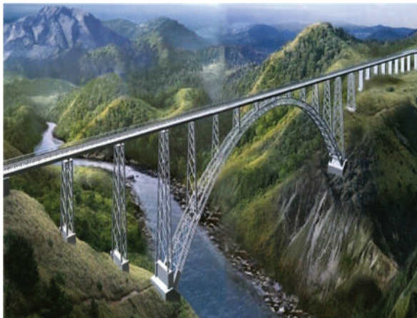
Photo: Artistic view of bridge being built across river Chenab
