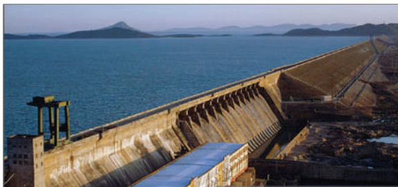
Figure: Perspective view of Hirakud dam
