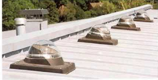
Fig. 4.64 Prismatic elements redirect the Sun's rays deep into the room, improving the uniformity of illuminance (left). Skylights in the form of light tubes can be up to 10 m long and conduct the light by multiple reflections several floors below (right) [28, 29]
