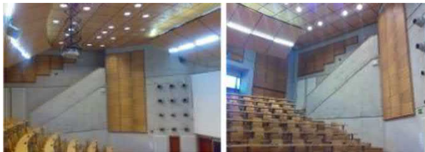
Fig. 5.44 In rooms with non-parallel walls, it is easier to avoid resonance (left). Sound absorbers ensure that the time difference between the moments when direct and indirect sound waves are detected is so short that sound monitoring is not disturbed. They should be installed on the ceiling and at the back of the room (right)
