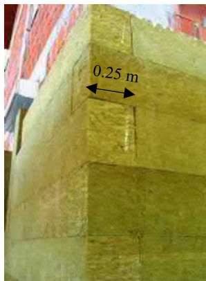
Fig. 1.35 Thick thermal insulation layer is needed to fulfil the criteria of permissible thermal transmittance U_{\max}
