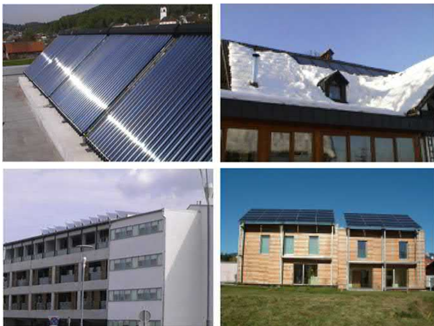
Fig. 2.23 Vacuum tube solar thermal collectors on the flat roof of a technology centre, flat solar thermal collectors on the roof of an inn (above), a solar thermal system for the heating of domestic hot water on the flat roof of a elderly-people's home, and a photovoltaic system on a two-family building. These technologies enable the on-site production of the heat and electricity needed for the operation of the buildings
