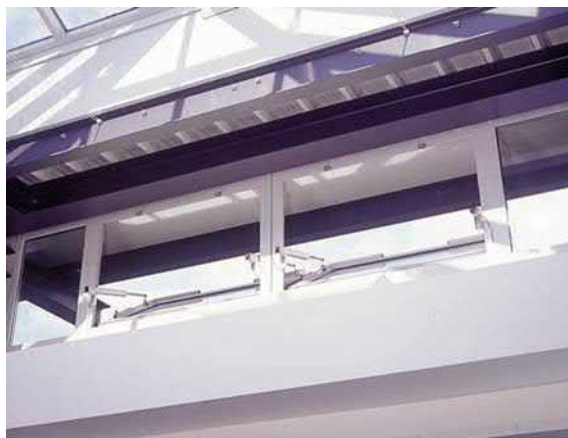
Fig. 6.29 Smoke flaps with automated opening mechanisms [24]
