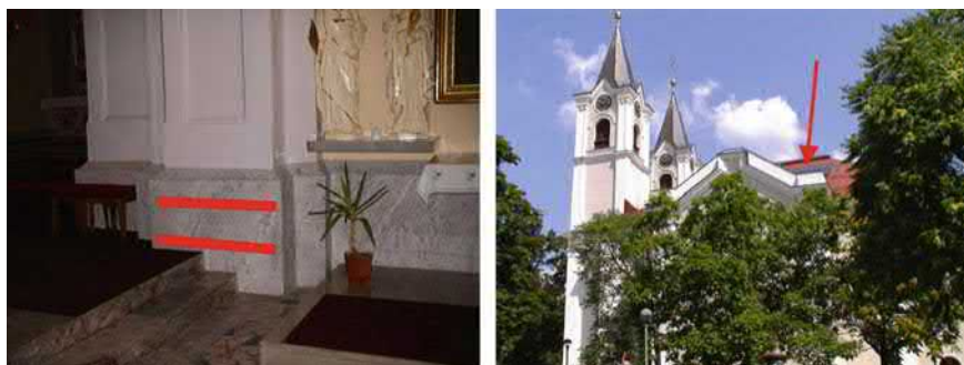
Fig. 3.18 Heating pipes were laid in two levels in the walls at the St. Peter and Paul church in Zagorje ob Savi, Slovenia. Water with temperature between 25 °C and 30 °C circulates the pipes all year long. The church has been fitted with a solar heating system to make the heating both energy and cost efficient [16]
