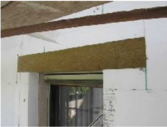
Fig. 6.15 Thermal insulation of residential buildings must have at least response-to-fire class B-d1. In the case of buildings taller than 22 m, the section of thermal insulation with response-to-fire class A1 or A2 must be applied with a width of at least 20 cm above the windows and doors and must be extended at least 30 cm beyond the edge of the window or door. Facades with an open air gap must be built with thermal insulation having response-to-fire class A1 or A2, s1, d0 to prevent the spread of the fire in the air cavity
