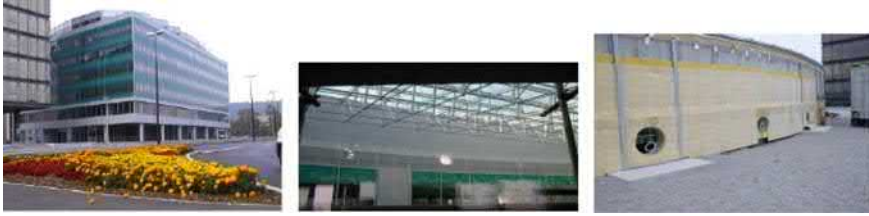
Fig. 6.31 Five fans are installed on top of a commercial building atrium (left) to extract smoke in the case of a fire (mid, left). Inlet openings with automatically controlled flaps are installed in the ground floor of the atrium
