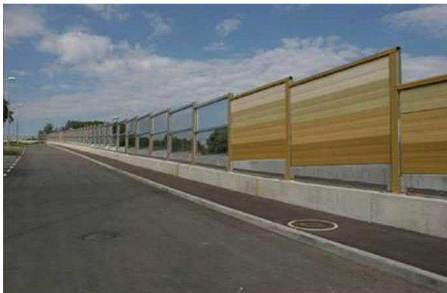
Fig. 5.24 Noise barrier along a road consists of a noise-absorbing part (panels with a porous material in the foreground) and a noise-reflecting part (glass panels) [10]
