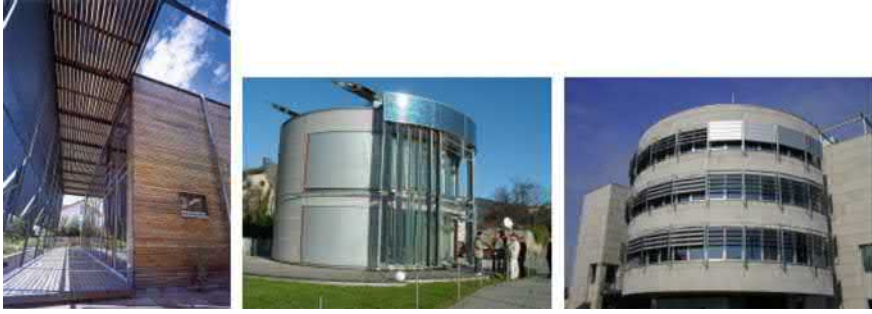
Fig. 1.57 Shading devices should have a high solar irradiation reflectance and must be offset from the façade, so they cool by circulating air on both sides and enable daylighting (left). Shades should be controlled by a building management system (BMS) (middle), nevertheless they must be designed so that the occupants can adjust the position of the shades to personal needs (right)
