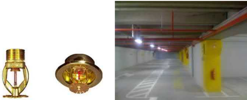
Fig. 6.25 Sprinkler heads; red fluid in the glass bulb indicate that the sprinkler system will activate at approximately 77 °C [23] (left); sprinkler system for automatic fire extinguishing in an underground garage; each sprinkler head covers approximately 20 m 2 , demanding a complex network of pipes for water supply (right)
