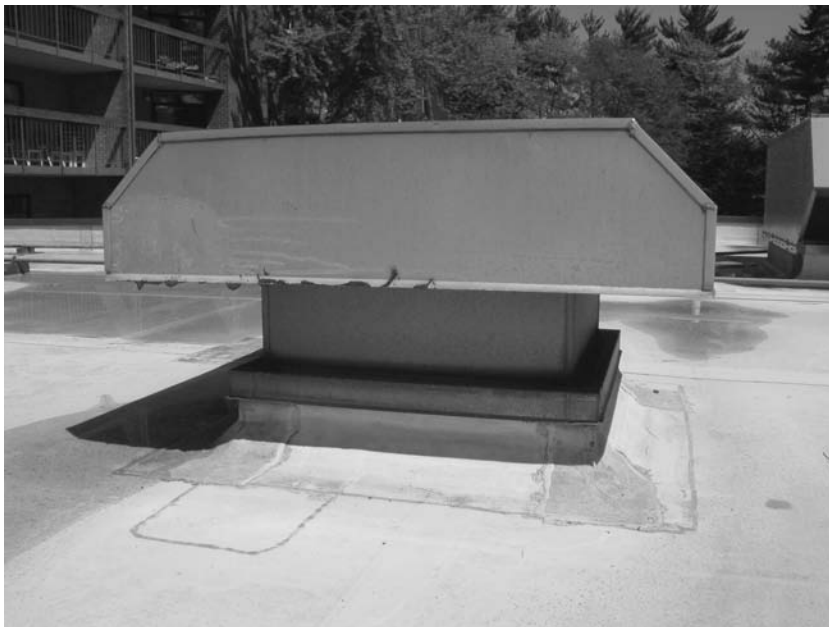
FIGURE 2-9 Typical intake/exhaust/relief air hood.
