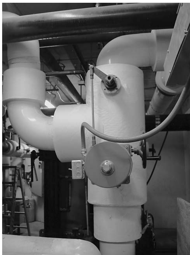
FIGURE 9-6 Photograph of a 3-way butterfly valve.
