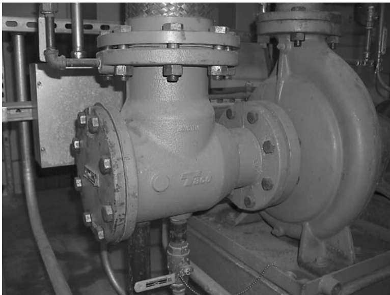
FIGURE 3-36 Photograph of a suction diffuser.
