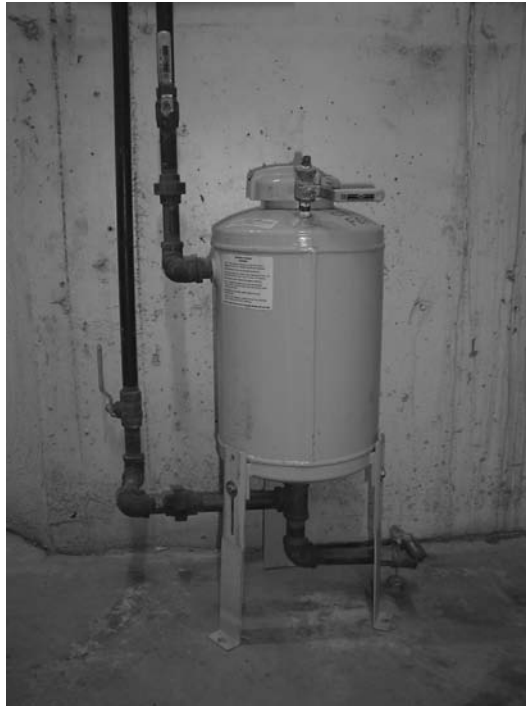
FIGURE 4-23 Photograph of a 5-gal shot feeder.
