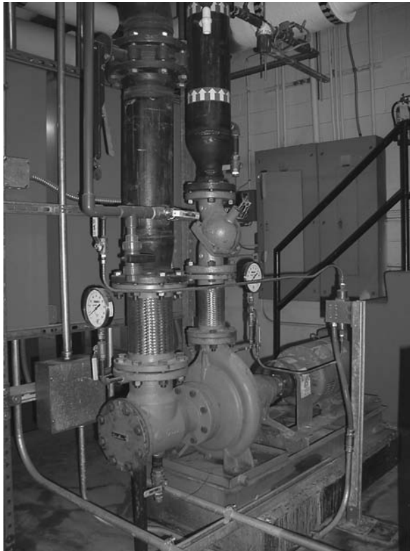
FIGURE 4-31 Photograph of an end-suction pump.
