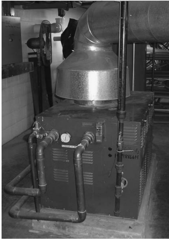
FIGURE 4-4 Photograph of a draft hood.
