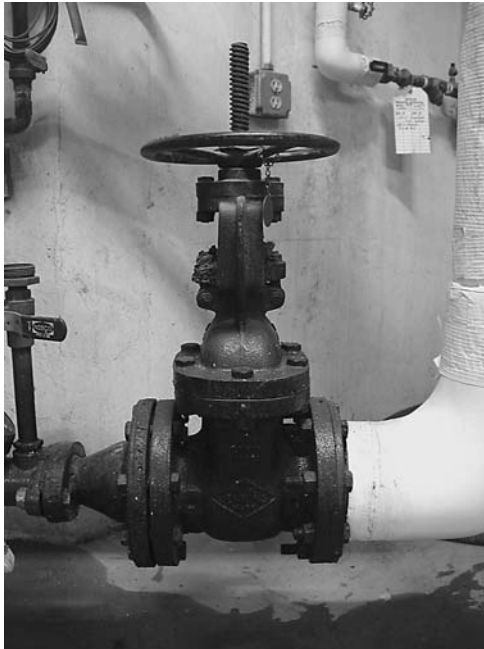
FIGURE 3-6 Photograph of a rising-stem gate valve with flanged ends.
